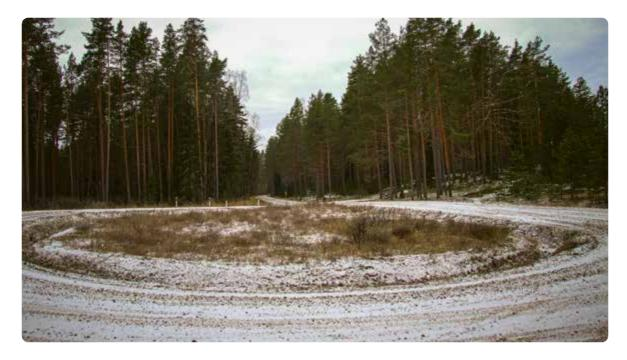
"Interim monitoring reports indicate that this type of structure is safe. After construction, a small amount of settlement occurs, which is related to the tension of the geotextile between the wooden piles, then the settlement of the road structure stops. Such a road structure could be used in the future in places where there are very low-level load-bearing soils and it is not possible to change the course of the road," concludes lvars Caune.
