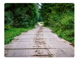
They also have the advantage of being re-usable, with each shield section likely to see service around ten times. Though forest shield roads are usually fairly short with a couple of hundred metres being a typical length, LVM used one as long as 880 metres beside the "Mežsargi" forest road in northern Kurzeme. ▲
